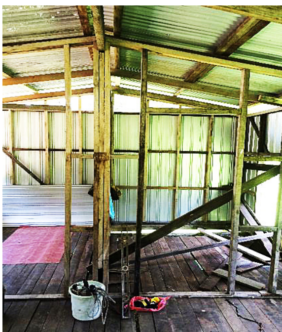
Figure 2: Timber frame home under construction in the rural region surrounding Madang.
