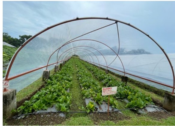
Tunnel/igloo structure, curved roof
