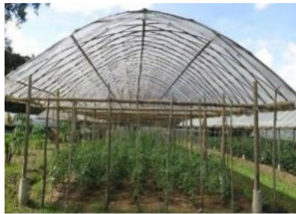
Modified curved roof system
