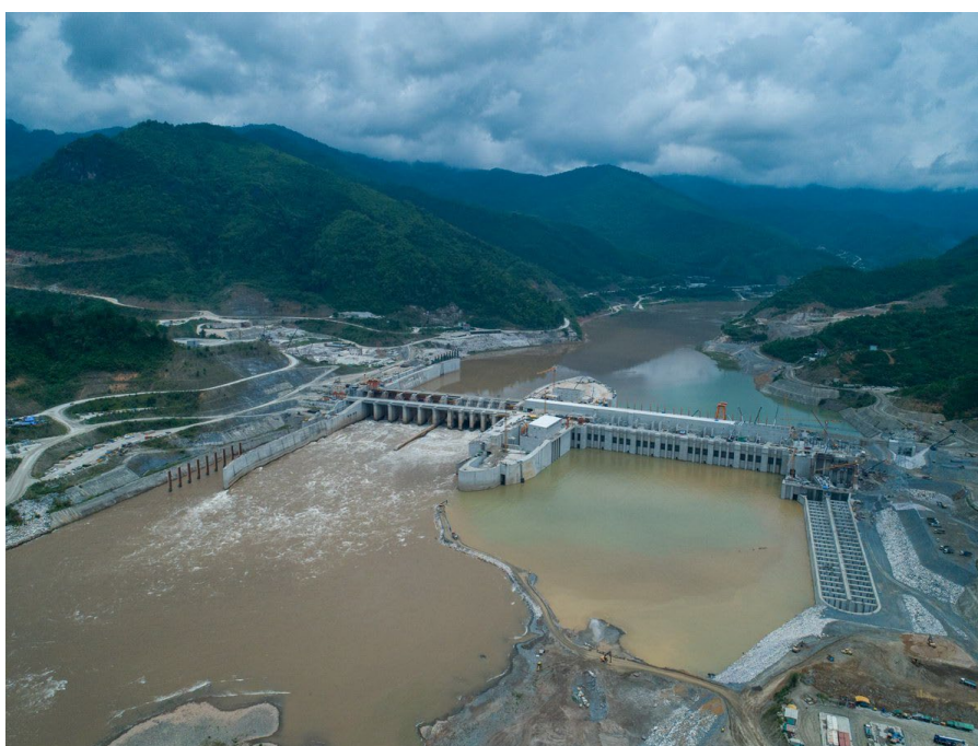
Figure 1. Aerial view of the Xayaburi Hydropower project looking upstream during the construction phase. The fish pass is located on the right-hand side of the HPP in this picture (source: unknown).
