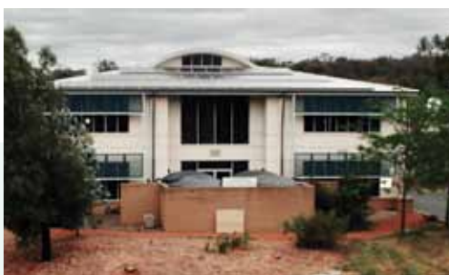
A bank of 48 solar panels was installed on the roof of ACIAR House in Canberra as part of ACIAR's Climate Change Initiative.
