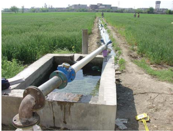
Figure 1. Experiment 1 — flowmeter and piped irrigation system with individual outlets to each plot
