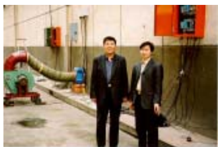
Preparing the control equipment in De Yang, Chengdu for demonstration during the training course field trip
