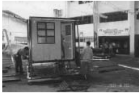
d. Workers installing accessories using simple carpenter's tools
