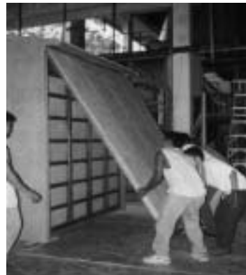
b. Trial run to check roof-to-case connection
