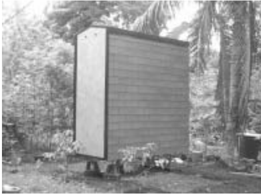
a. The emergency shelter is delivered to the site in a rigid case. The rigid case is mounted on adjustable prefabricated footings.
